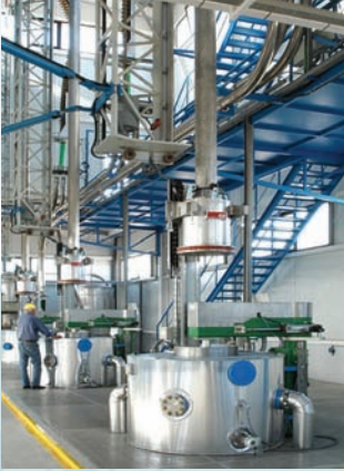
Cork purification plant
