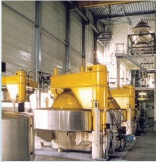
Tea decaffeination plant Supplied under Schoeller-Bleckmann
