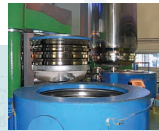
Edible oil extraction plant
