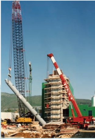
Coffee decaffeination plant Supplied under Schoeller-Bleckmann
