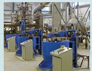
Supercritical fluid extraction Industrial plant, 3 x 850 l/550 bar
