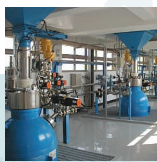
Rice treatment plant
